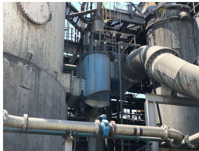
Installation on bypass system
